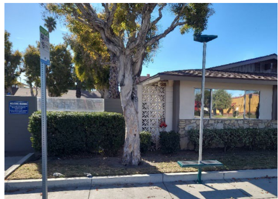
Bench and Solar Lighting installed at Gonzales & Ventura Road
